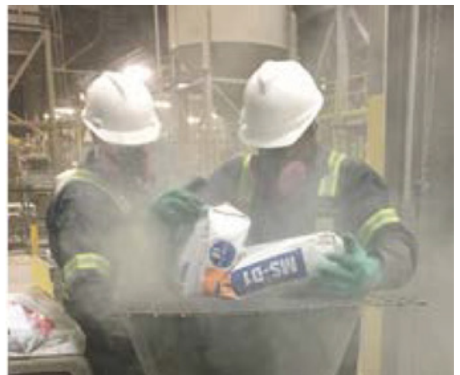
Fig. 8: Dry-mix shotcrete without any additives.
