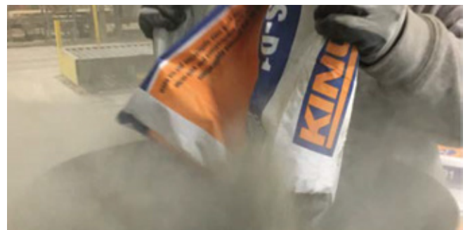
Fig. 2: Case 2: High concentration of dust emitted when pre-packaged dry-mix is emptied into the material hopper of a dry-mix shotcrete machine.
